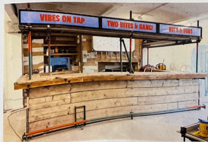
Interior - in progress
